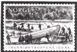
Construction of pontoon bridge, Nkr4.60 blue
